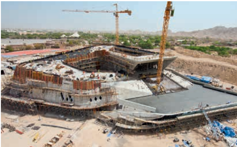
Fig 2 Desert learning center construction site, Al Aïn - Abu Dhabi
