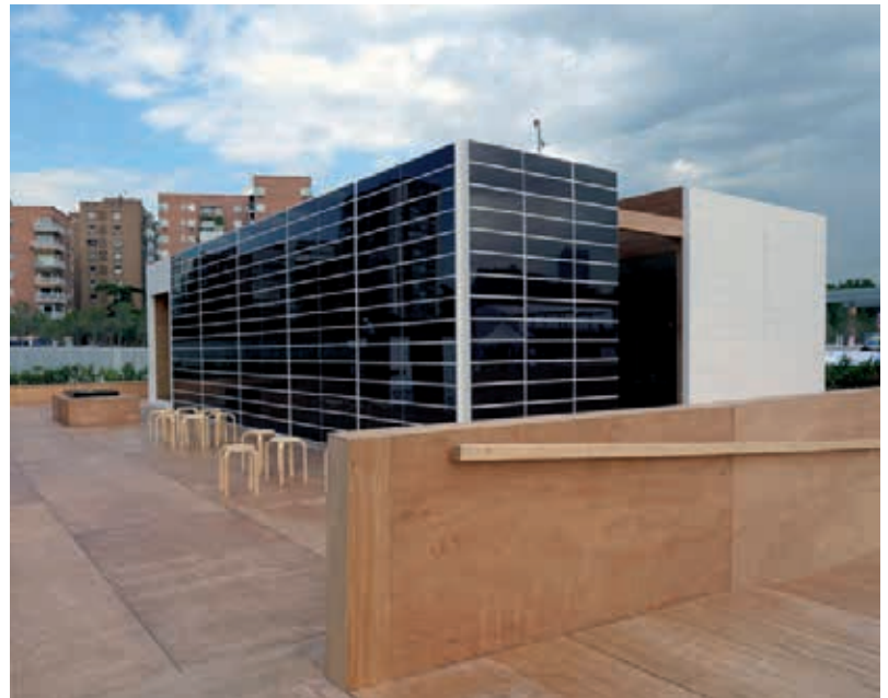
Fig 3 Ventiladed PV façade. Built for Solar Decathlon Europe 2010
